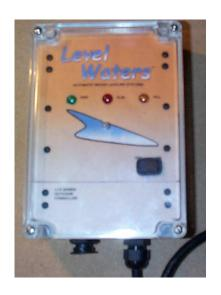
Make sure that the power switch is in the OFF position. Remove clear front cover. Remove the four screws in the access panel on the controller. Using ½" liquidtite conduit, run 14/2 Romex through the liquidtite panel connector and wire to power terminal block as shown in figures 1 & 2. Run control and sensor cables through the 3/8" watertight fitting and wire to control terminal block as shown in figures 1 & 2.
