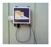
Connect the control cable WC-101 to the 6-prong jack on the FV-701 valve unit in the same manner as the sensor cable above. Install third #6 screw in the bottom tab and tighten all valve mounting screws.
