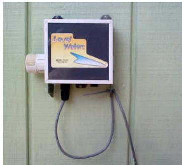
Connect the control cable WC-101 to the 6-prong jack on the FV-701 valve unit in the same manner as the sensor cable above. Install third #6 screw in the bottom tab and tighten all valve mounting screws.
